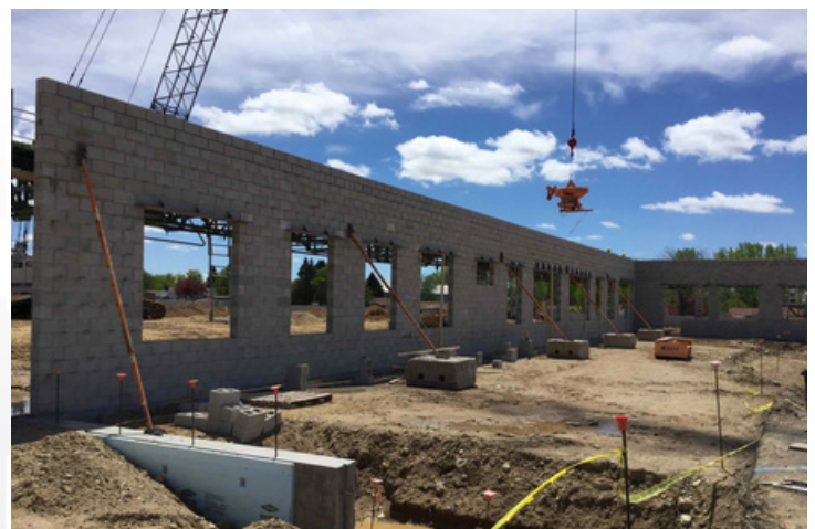
Block Walls for the Addition
