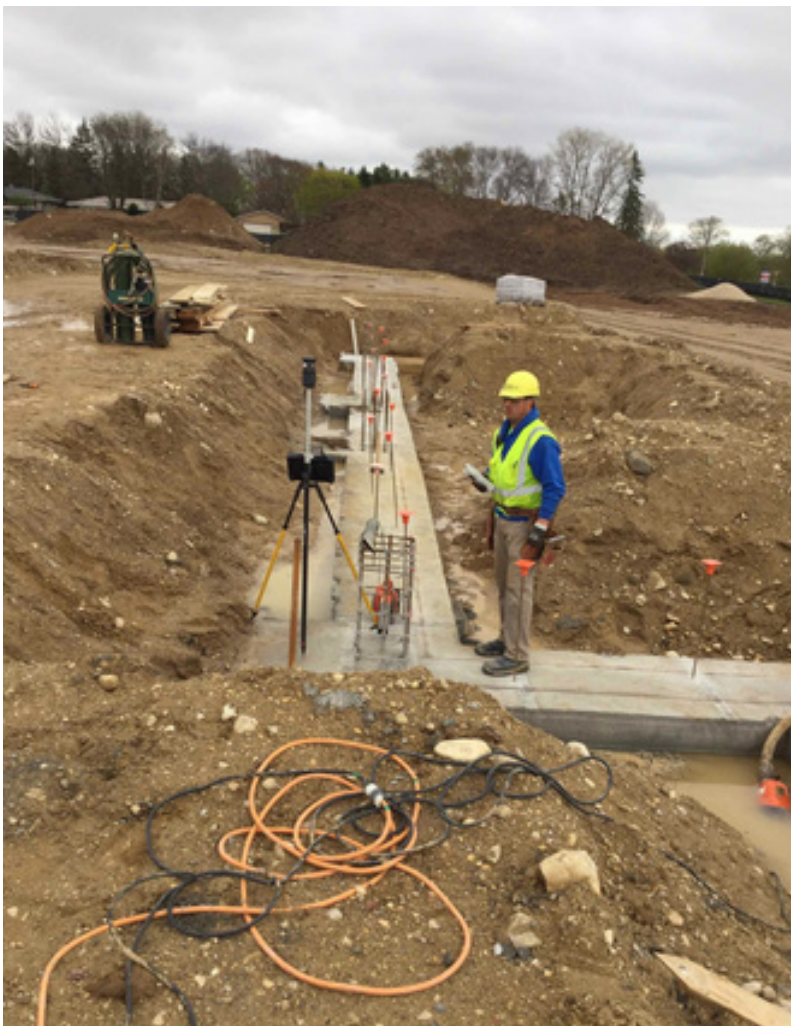
Recording Final Elevations for Foundation Wall Preparation
