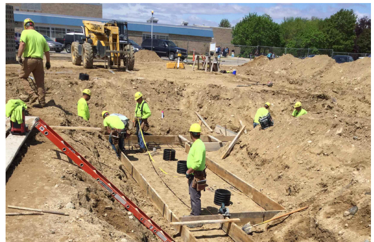
Footing Preparation for the Addition
